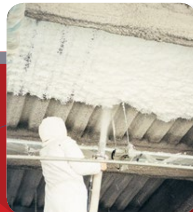
Non-combustible Monoglass applied over fireproofing, University of California
