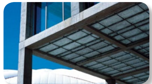
Soffit application to insulate occupied space above
